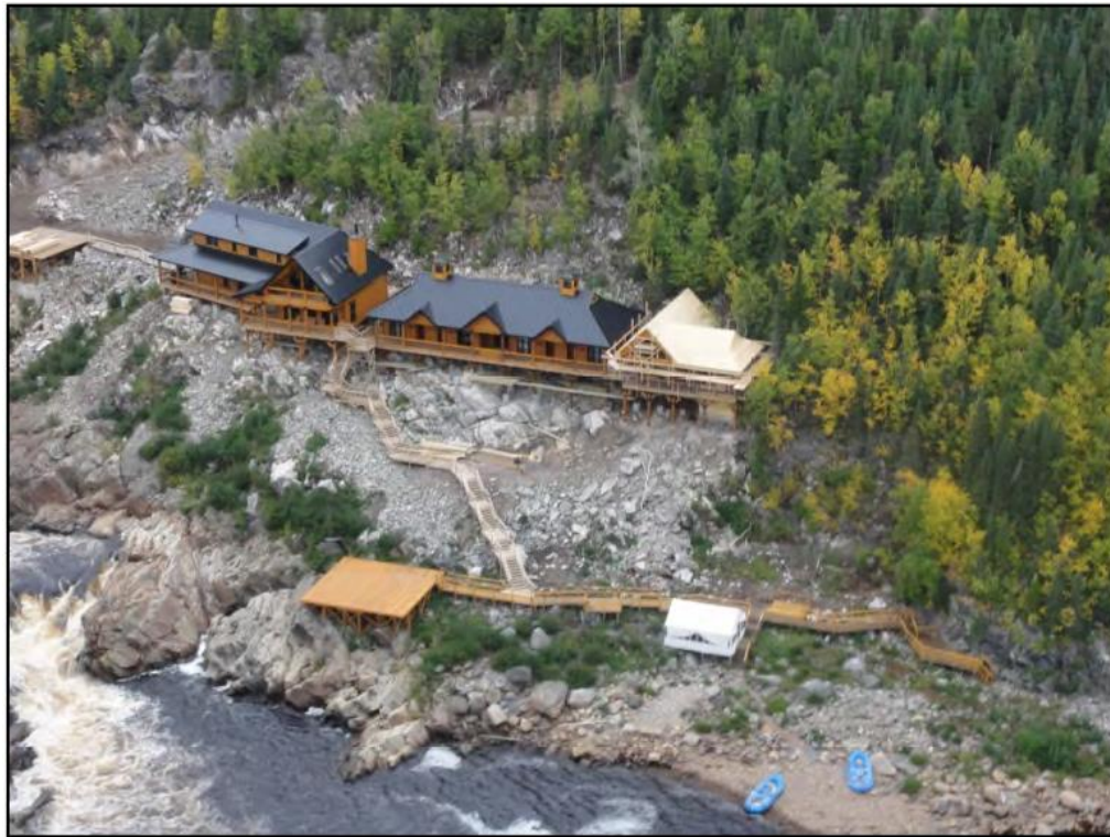
Figure 4: St. Lewis River Lodge
